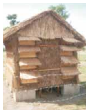
Figure 2. Improved Naturally Ventilated Storage Structure (INVSS)
